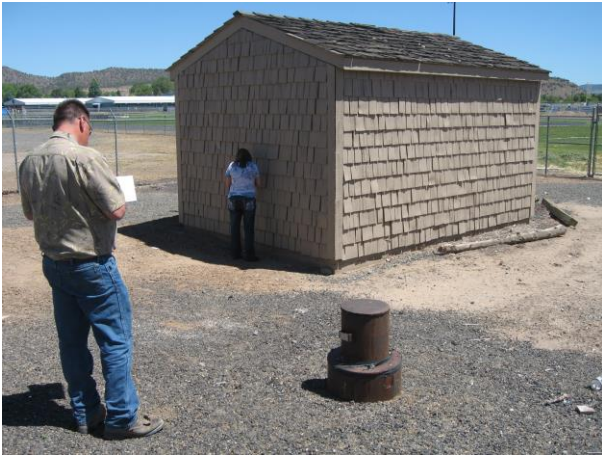
Photo 6 – Unused well next to Stadium Well control building.
