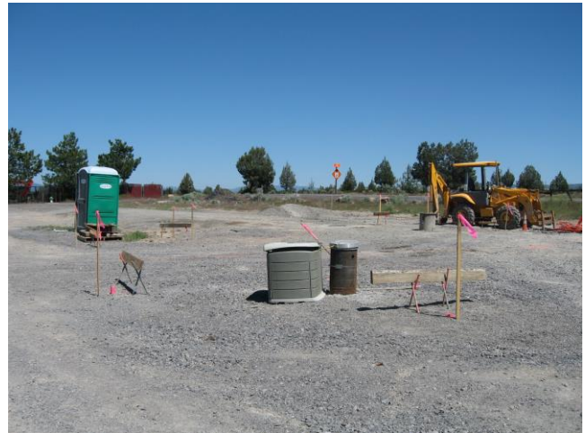
Photo 27 – New Airport Well 3 being constructed.
