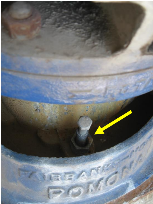
Photo 17 – Improve seal old down-hole chlorination openings for Yancey and Lamonta wells.
