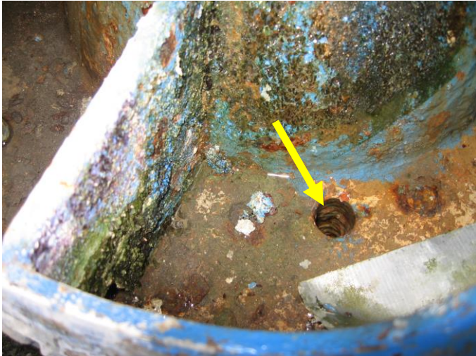
Photo 16 – Seal hole on pump platform into Yancey Well.
