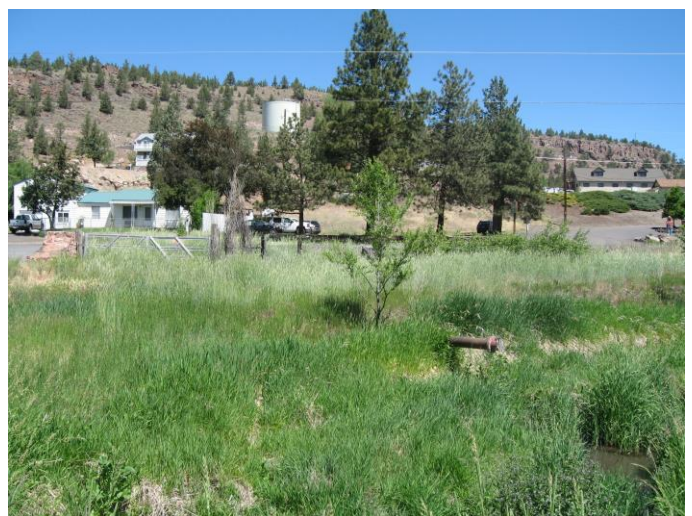
Photo 5 – Barnes Butte Reservoir screened overflow piping to canal.
