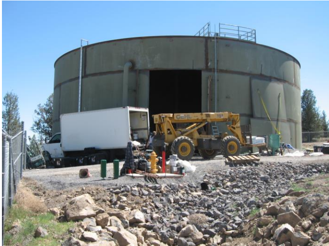
Photo 25 – New reservoir under construction next to Airport Reservoir.
