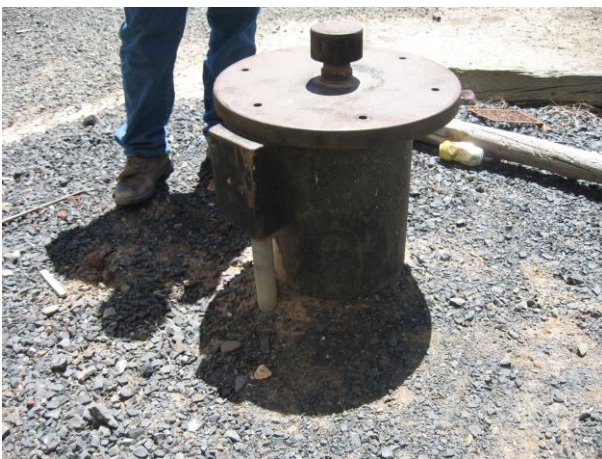
Photo 7 – Stadium Well on other side of control building.
