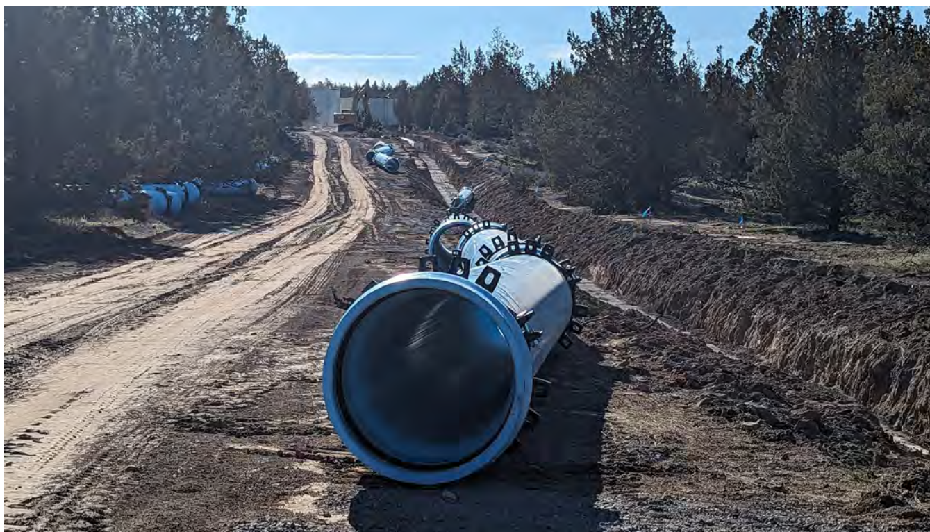
Water resiliency project in April 2024
