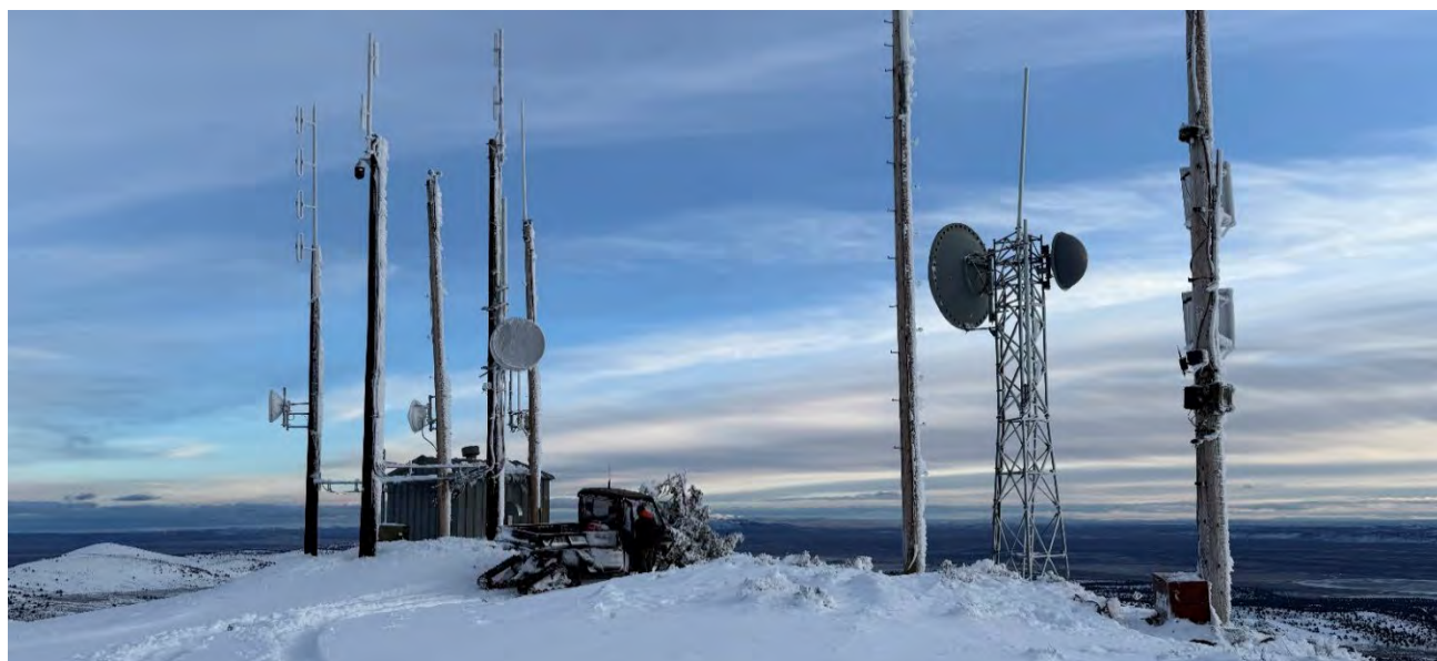
IT performs tower work in December 2024.
