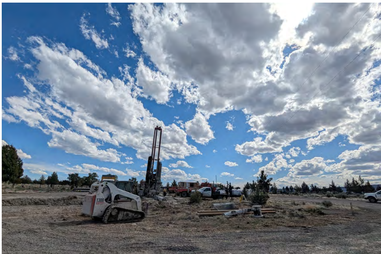
Well drilling in March 2025
