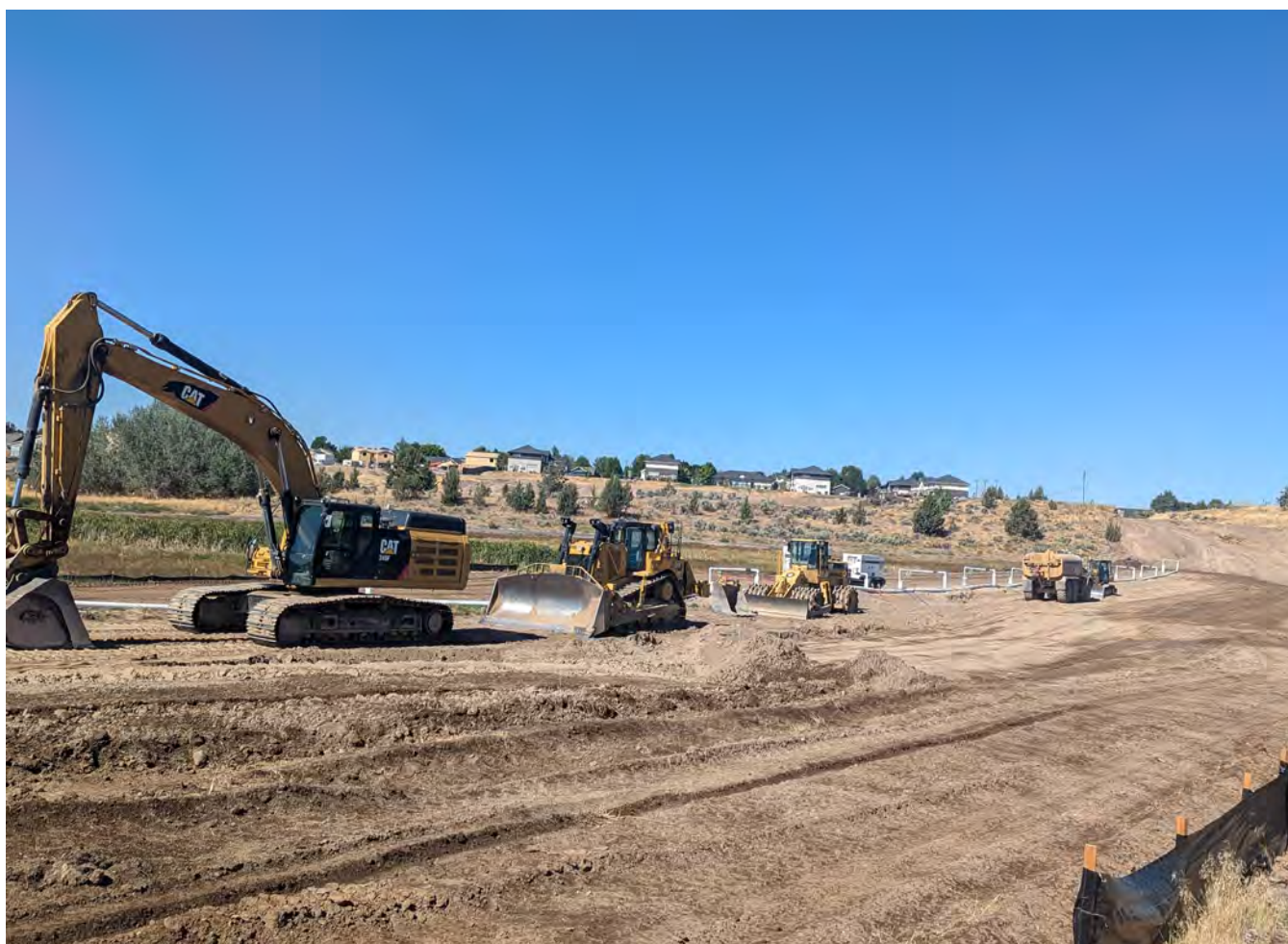
Combs flat extension project in August 2024
