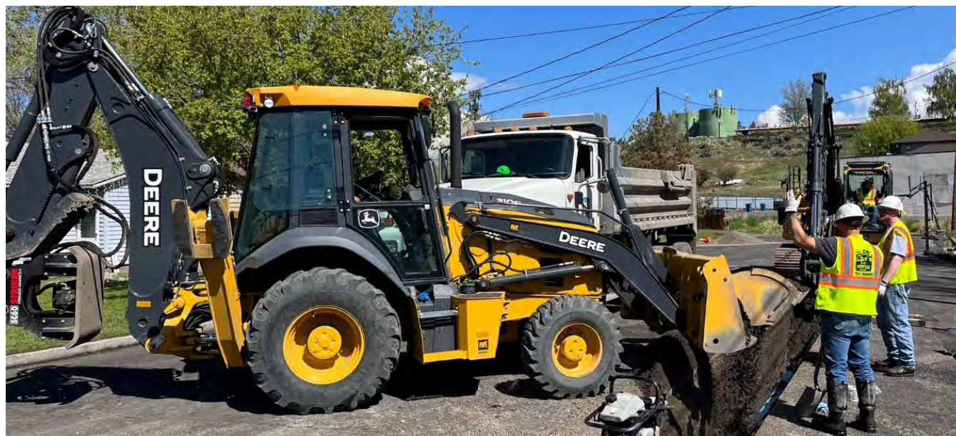
The Dunham waterline project in August 2023
