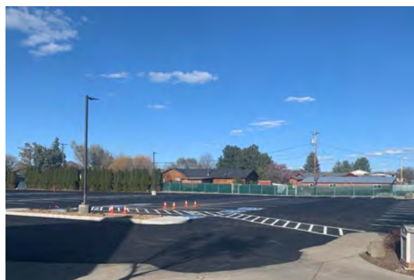
Meadow Lakes Parking Lot Paving in May 2024
