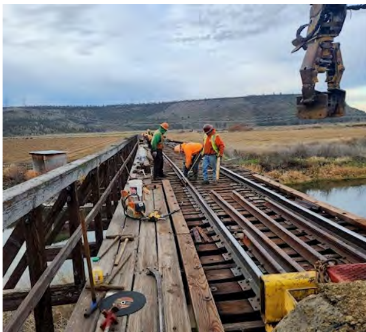
Railroad Bridge work in progress during December 2023
