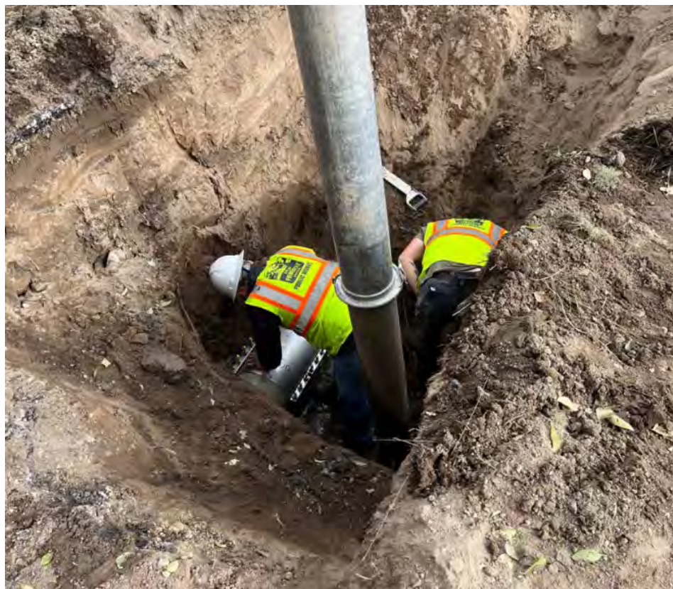
Utility Line work being done in BN 25
