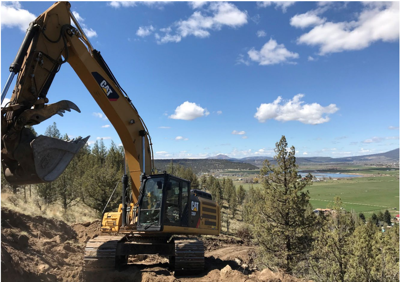
Contractors working on the Airport Industrial Park Utility project in 2019
