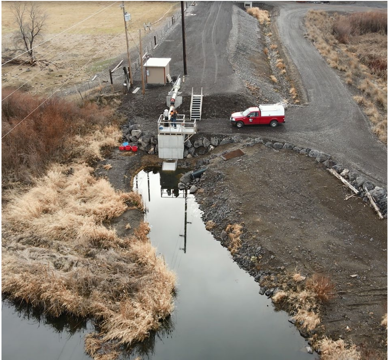
Newly constructed fish screen off the Crooked River
