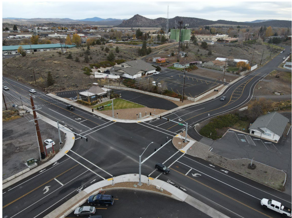
Completed realignment of the intersection of 10 th /N Main in 2021
