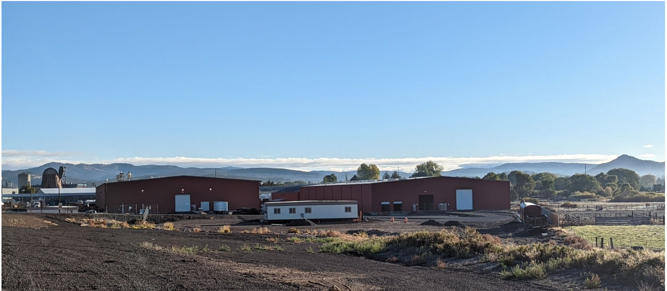
A view of the Freight Depot including its new office in October 2022
