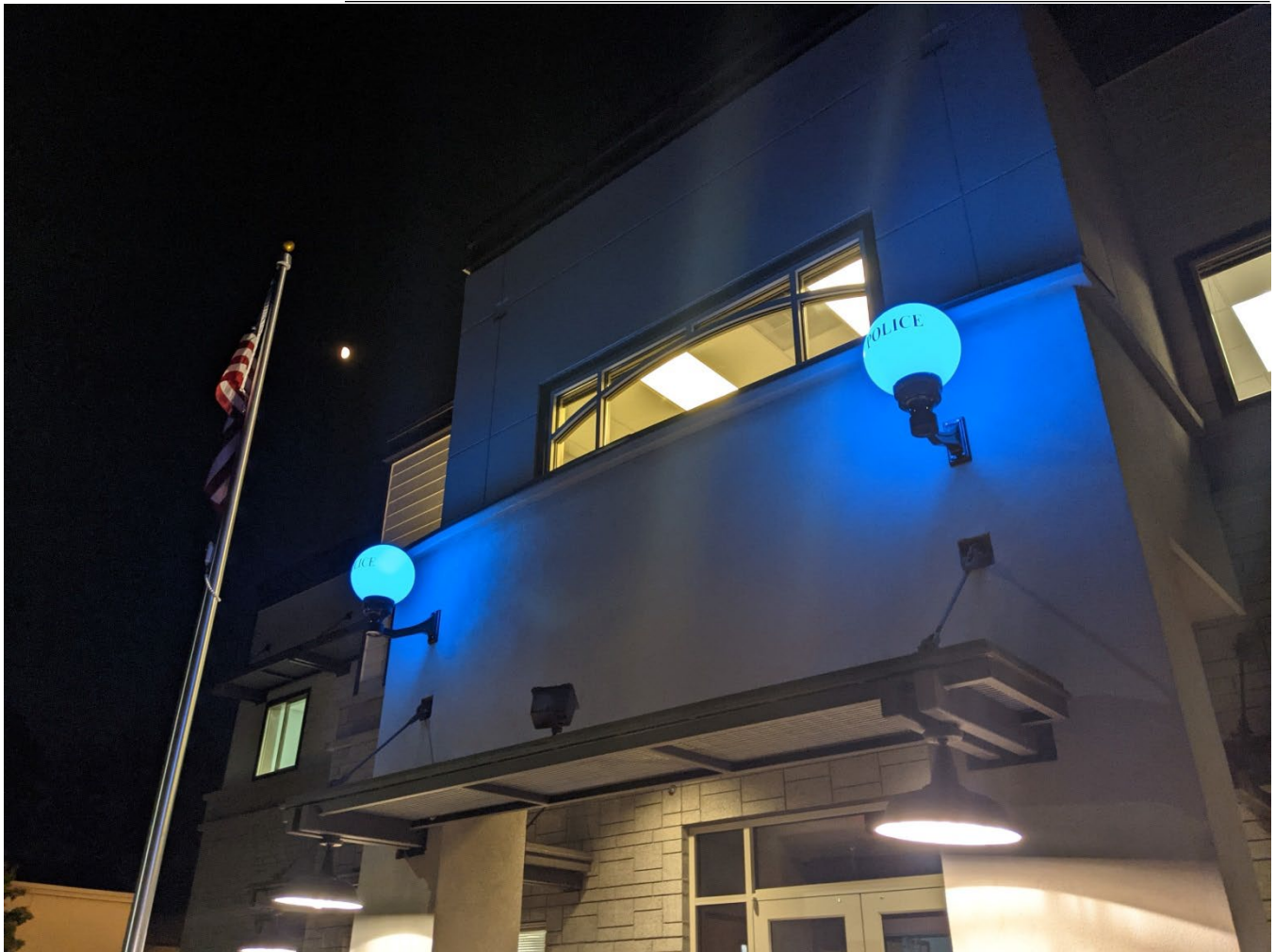
Both the Prineville Police Department and Crook County 911 fully moved into the new public safety facility (pictured above) at the end of FY 21
