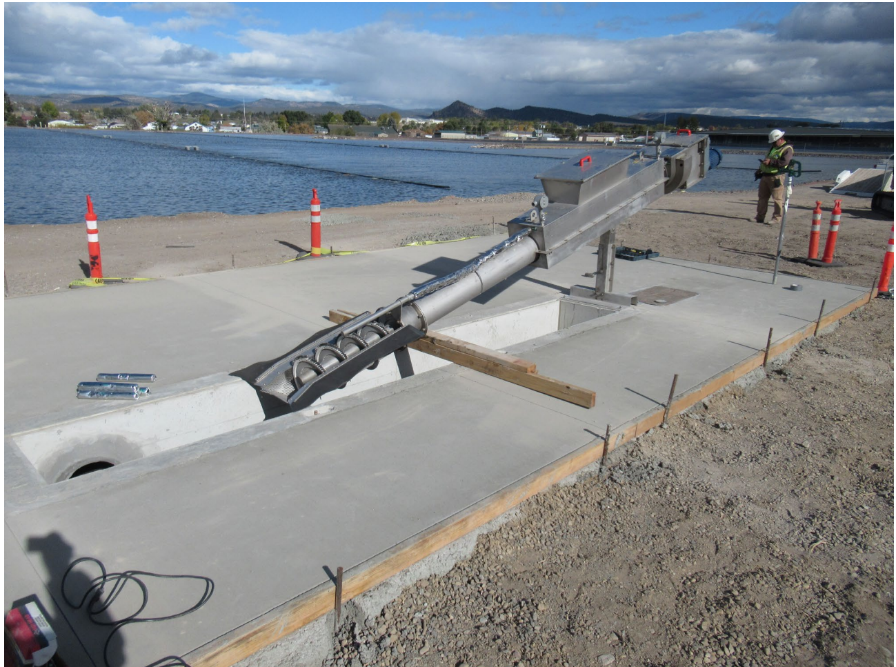
Wastewater treatment plant screen improvement done in April 2020
