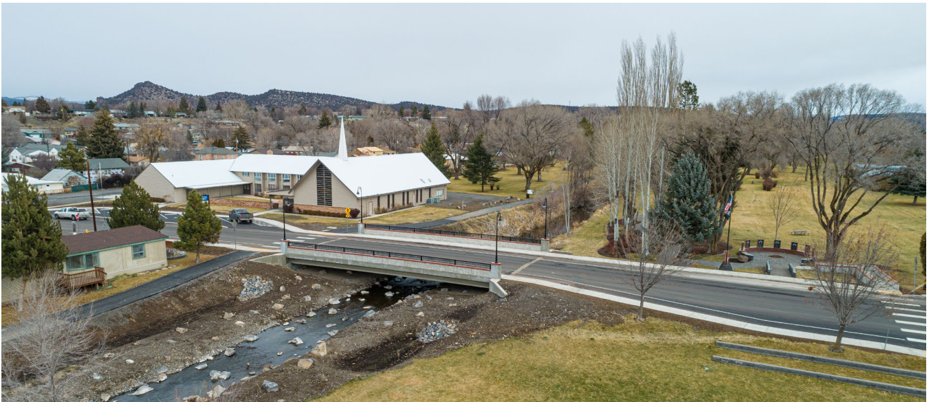
New Elm St. Bridge completed seen in early 2020 after its completion
