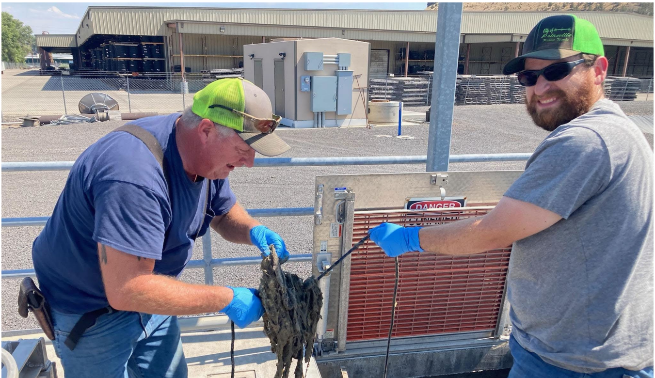
PW employees working at the wastewater treatment plant in 2023
