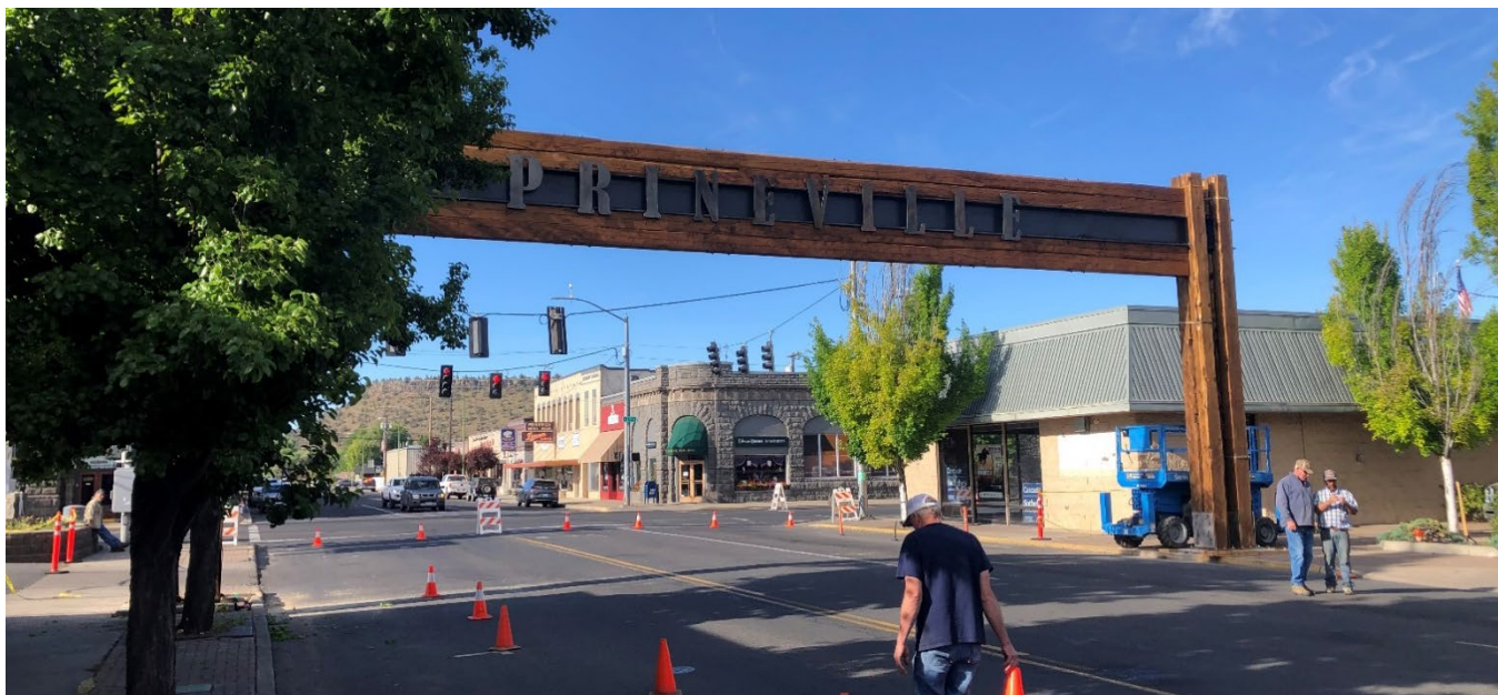
Downtown arch being installed in June 2022
