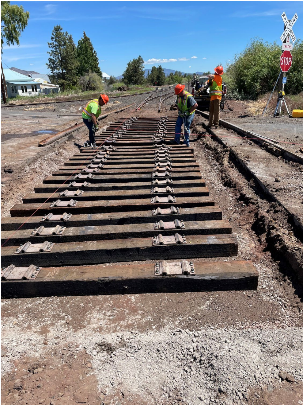
Laying down new cross-ties at a railroad crossing in 2023
