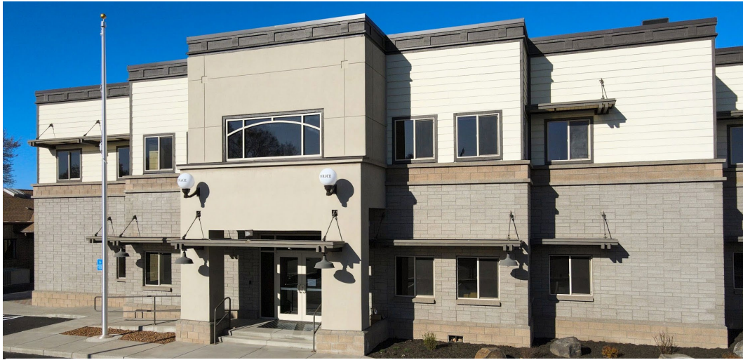
The Prineville Police Department and 911 Dispatch Center at 1251 NW Elm St.
