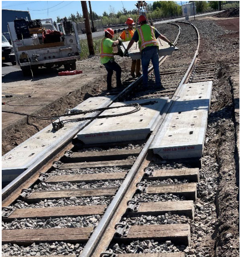
Railway crossing work completed in 2023
