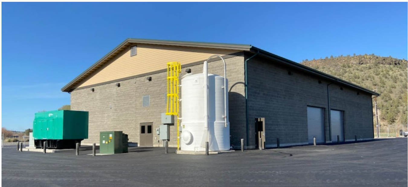
New ASR building constructed in FY 21
