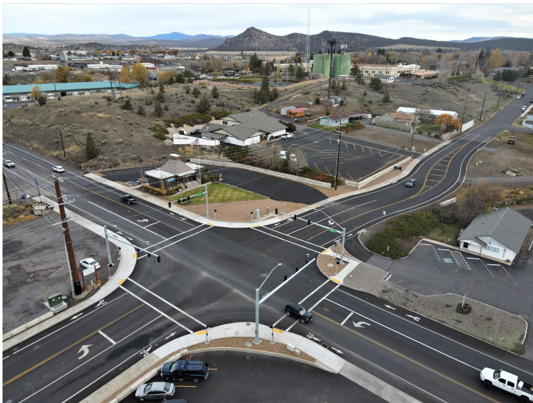
Completed realignment of 10 th and Main Street in FY 22
