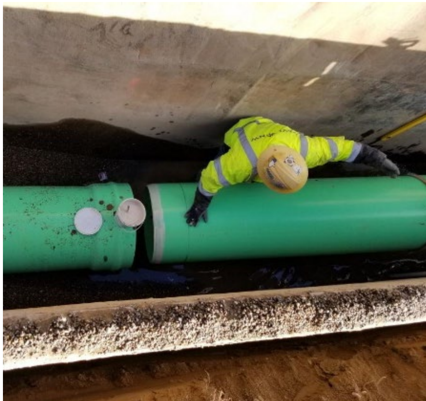
Waterline installation project from BN 21
