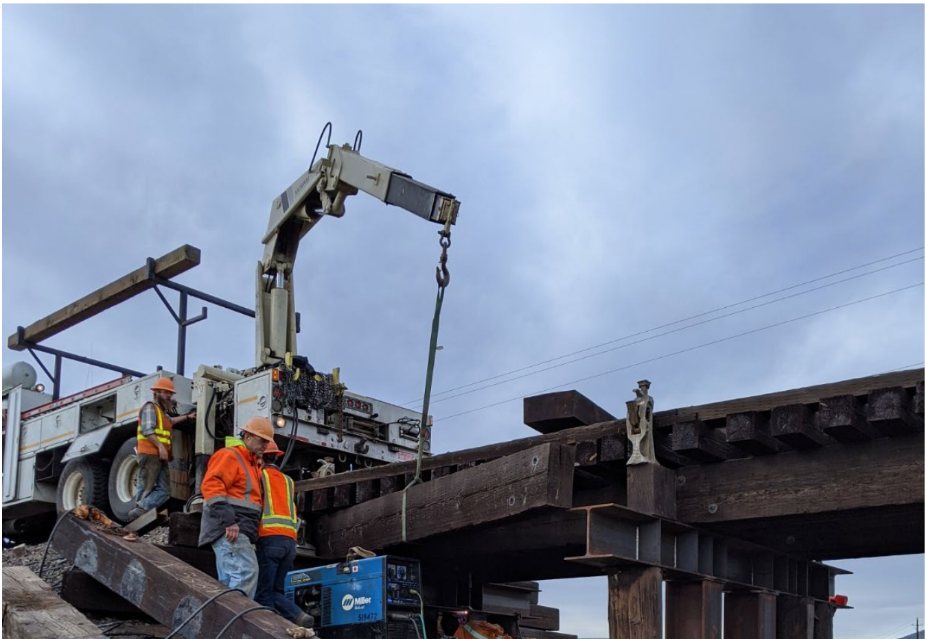
Contractors work on the Madras Highway Bridge in January 2020
