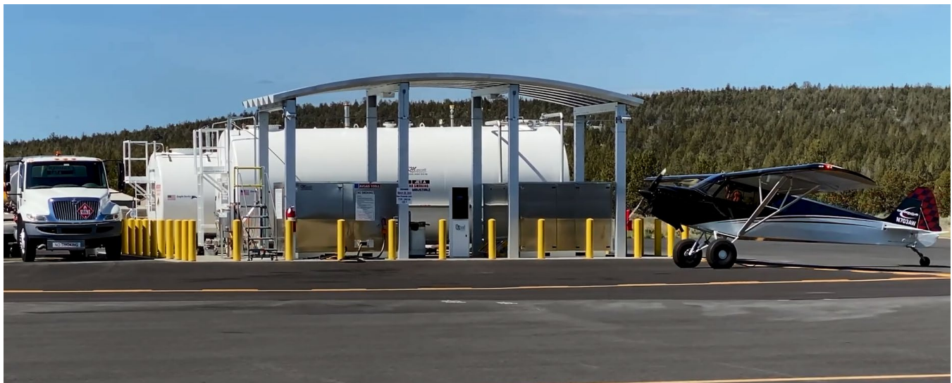
New airport fueling system completed in BN 21
