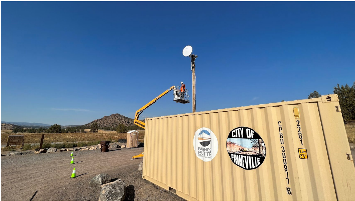
IT Department installing a link at the Barnes Butte Recreation Area
