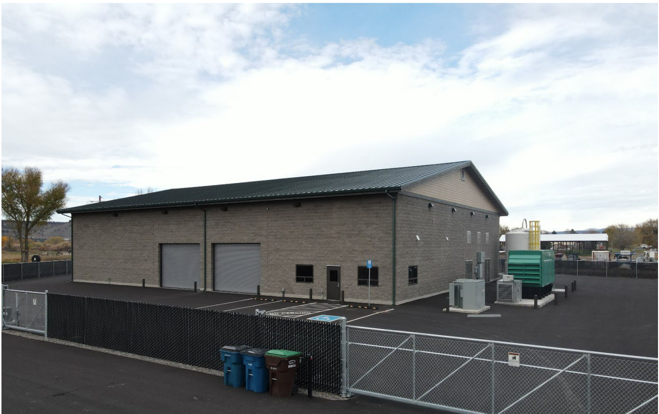
Completed ASR building as seen in November 2021
