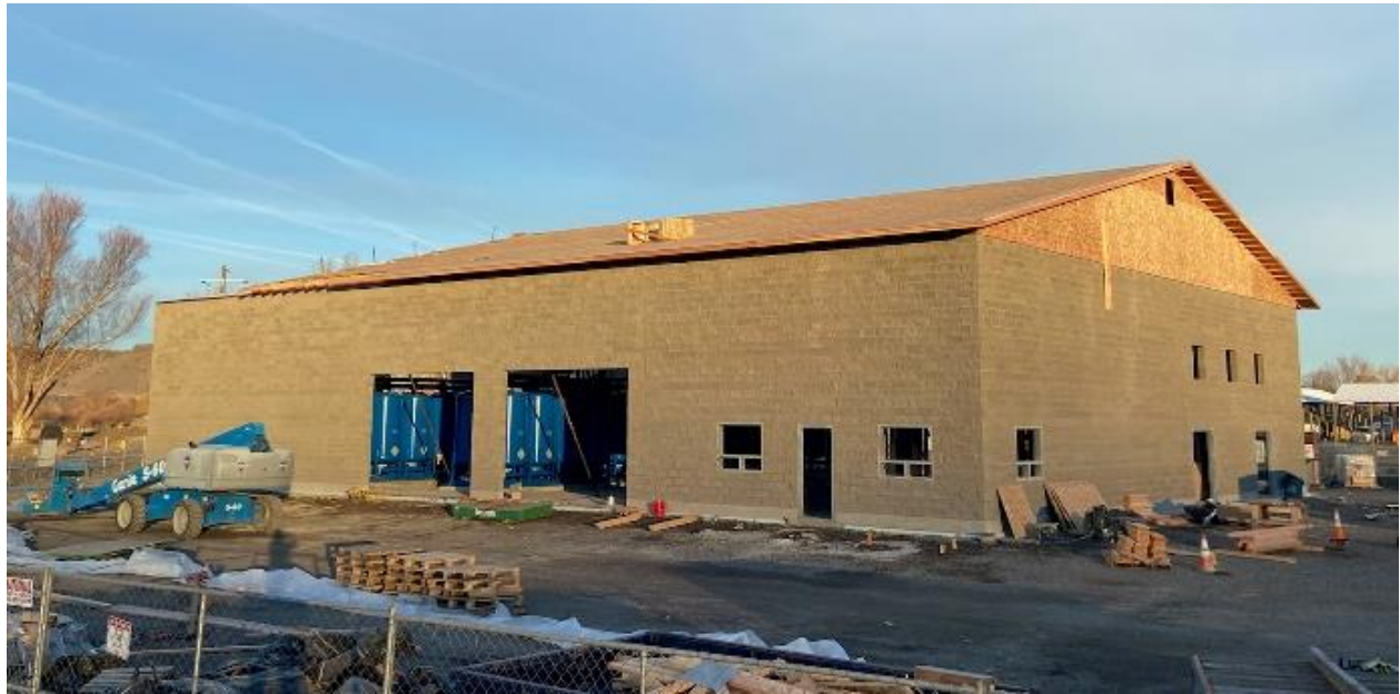
Second quarter progress of the ASR building.
