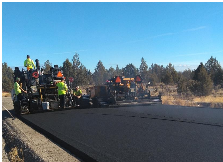
Helibase paving at the airport that took place during the second quarter.
