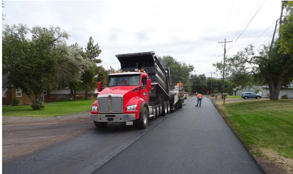
Paving a residential street in September 2017
