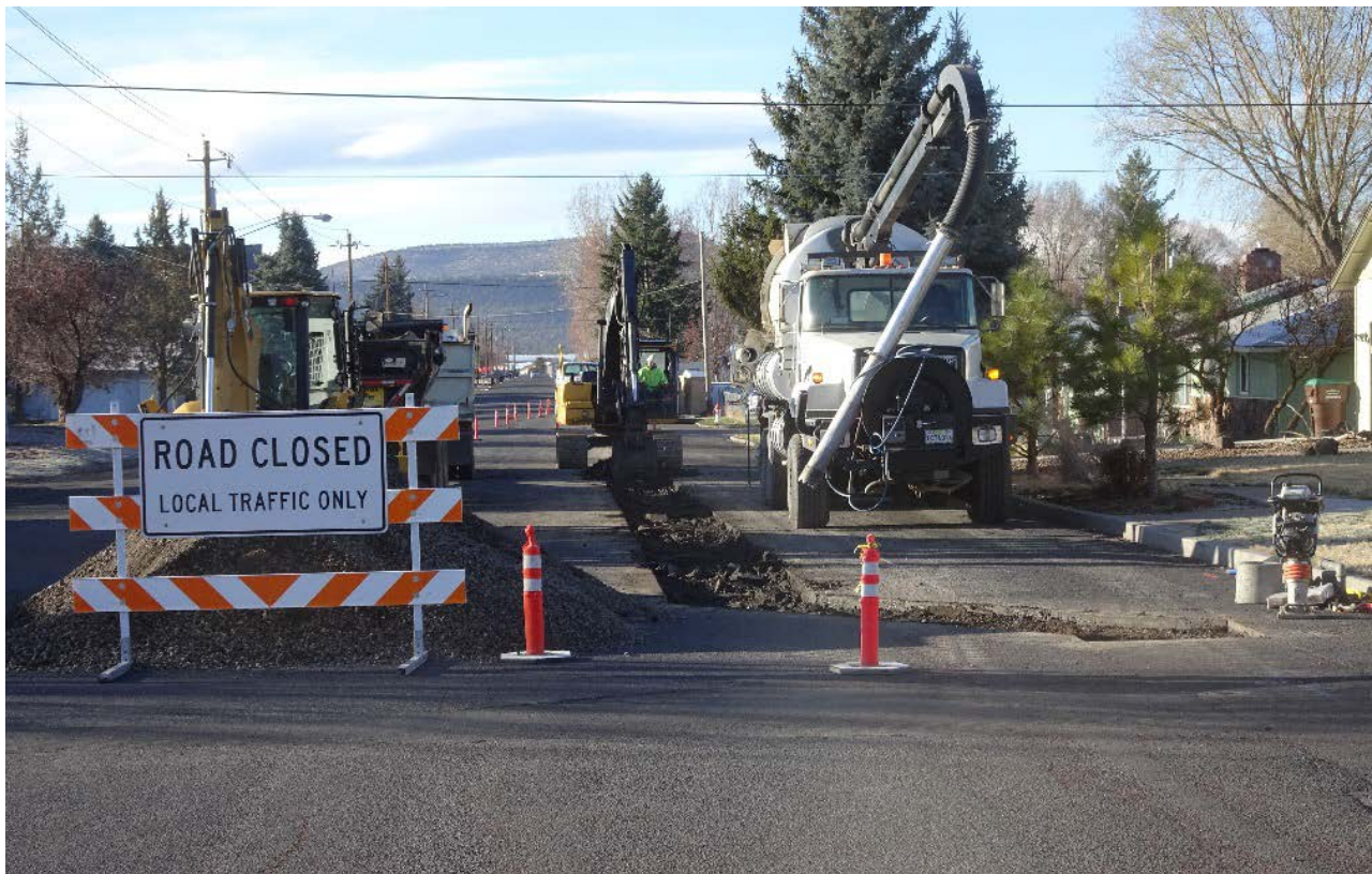
Work on the SE Fairview water line replacement in March 2018
