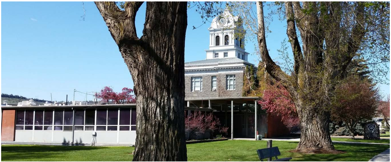
The Police Department and Dispatch Center will move out of its current location at 400 NE 3 rd St. in 2019.
