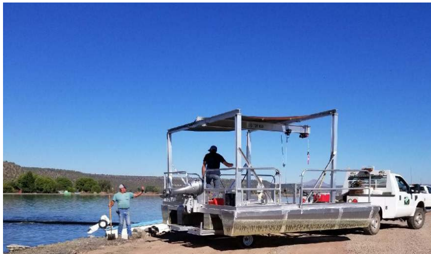
Staff moves a boat around the wastewater treatment plant to conduct work in July 2018.
