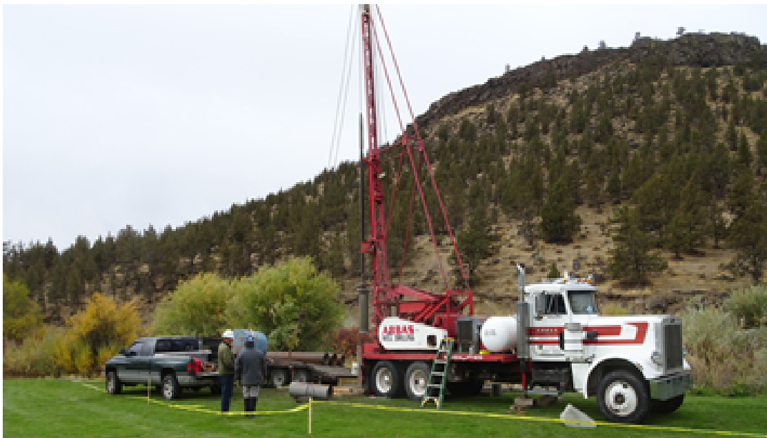
Drilling for the ASR project in October 2017
