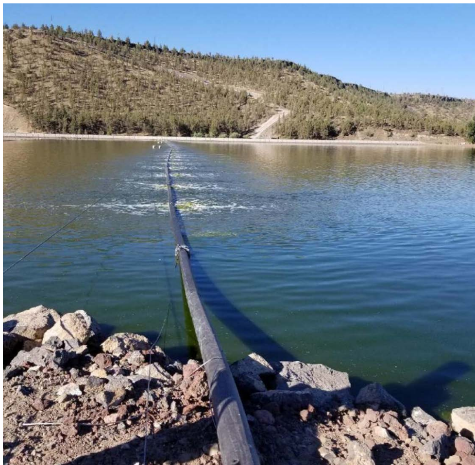
Wastewater treatment pond aeration maintenance was done in the summer of 2018.
