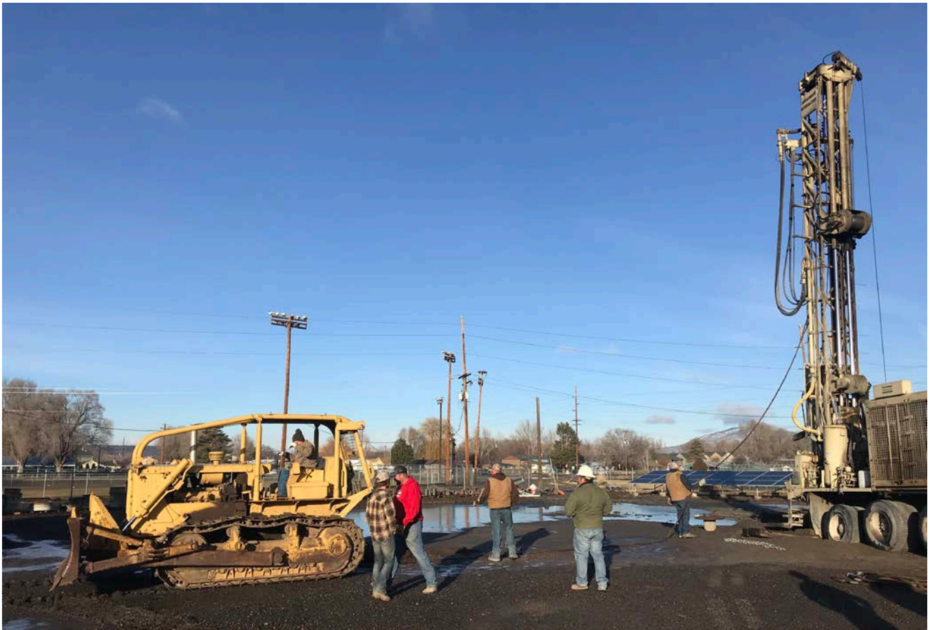
Public Works crew and contractors work on Yancey Well in December 2018
