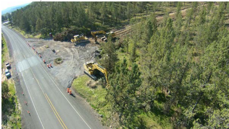
Equipment works on trenching up the hillside in April 2018
