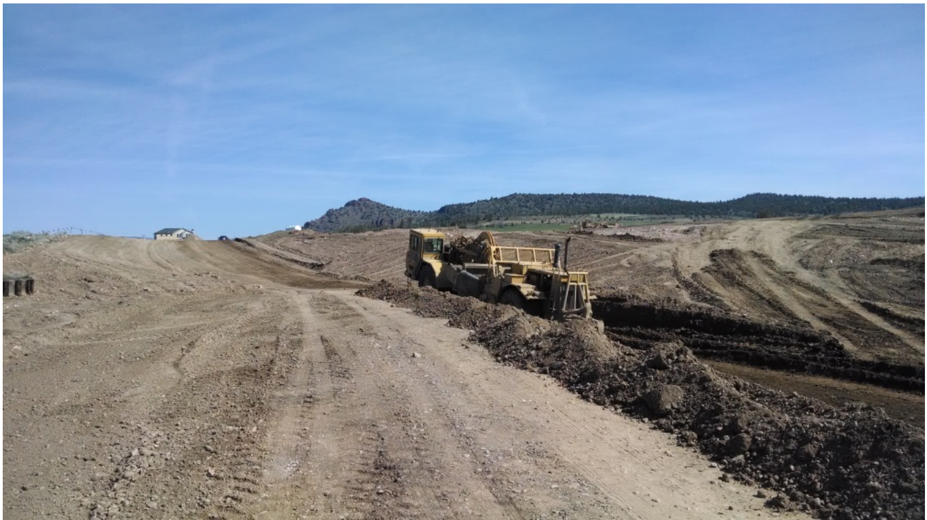
Road work starts to support the new school, Barnes Butte Elementary.
