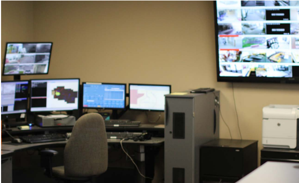
The 911 Dispatch Center after improvements were completed in 2014.
