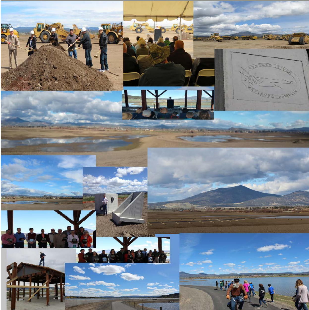
A sample of the progress of the Crooked River Wetland Project from its groundbreaking, construction and grand opening in 2017.
