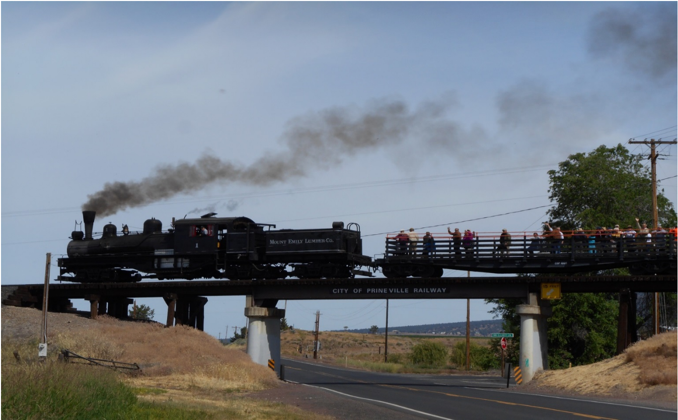
The Mt. Emily Shay giving passengers a ride over a bridge on Madras Highway.
