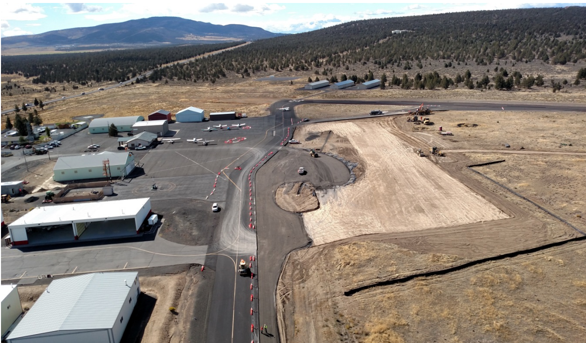
An aerial view of the construction at the Prineville-Crook County Airport.
