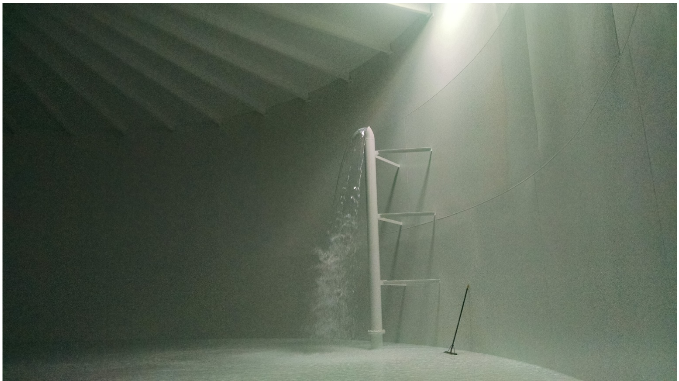
Filling Airport Tank #2 after its completion in 2014.
