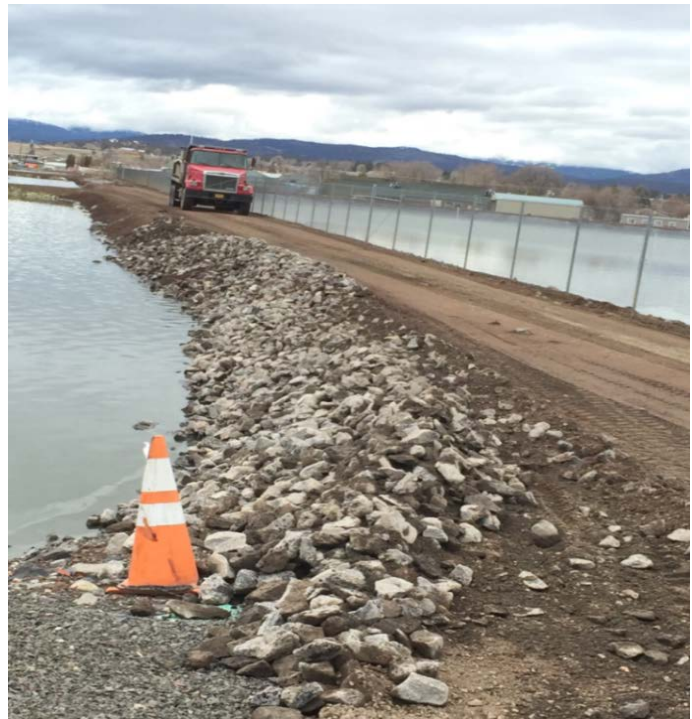
The Transportation Department widening dikes at the Wastewater Treatment Plant.
