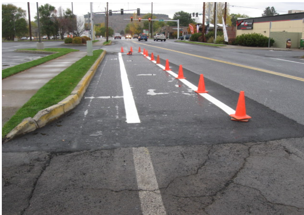
The start of bike lane restoration on NE Combs Flat Road.
