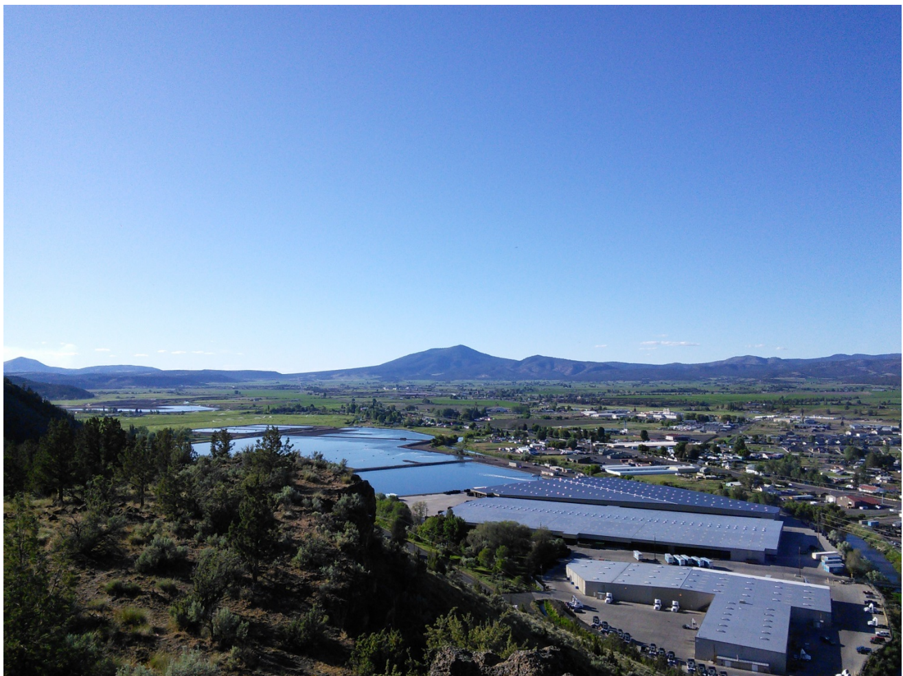
Looking over the wastewater treatment plant ponds on a sunny day in May 2016.
