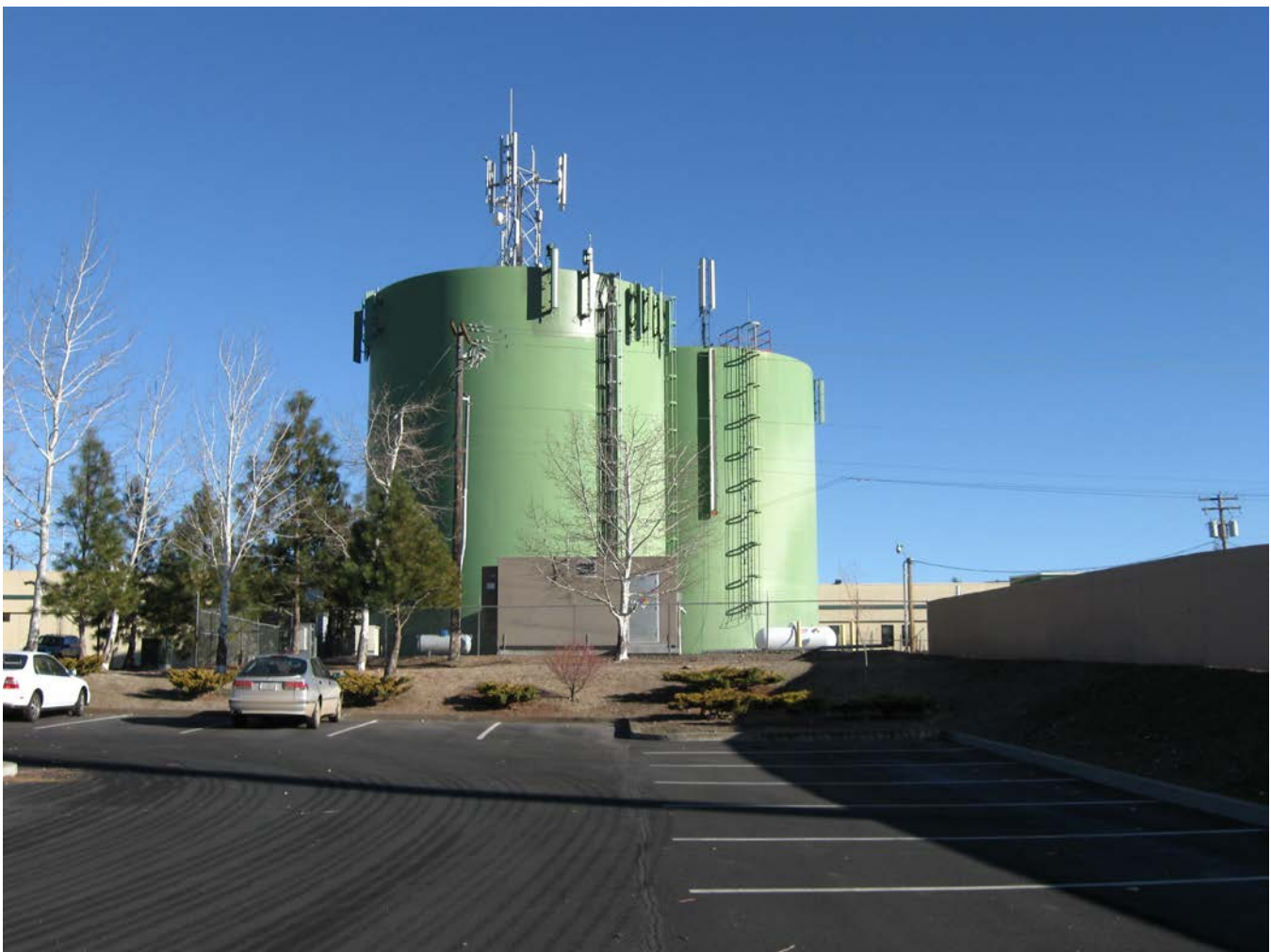
Two water tanks near the old Pioneer Memorial Hospital.
