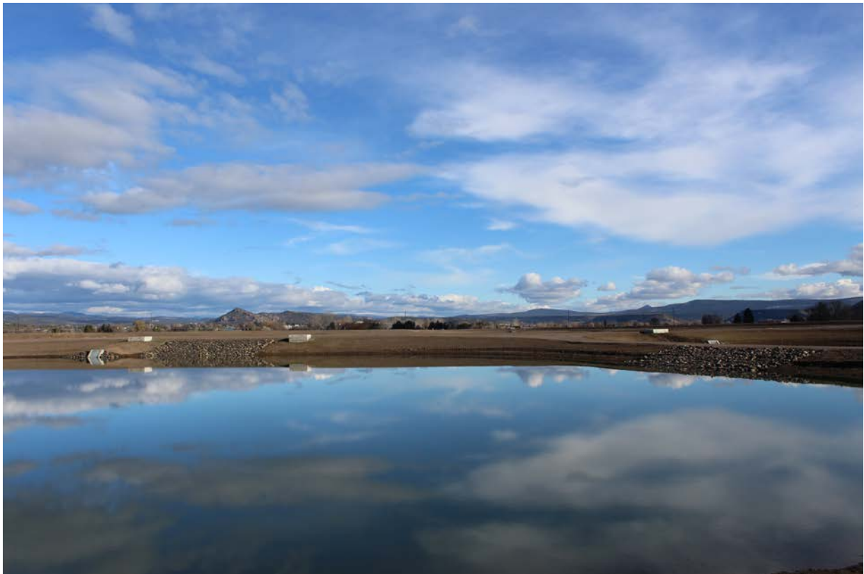
The Crooked River Wetlands Complex during construction in November 2016.
