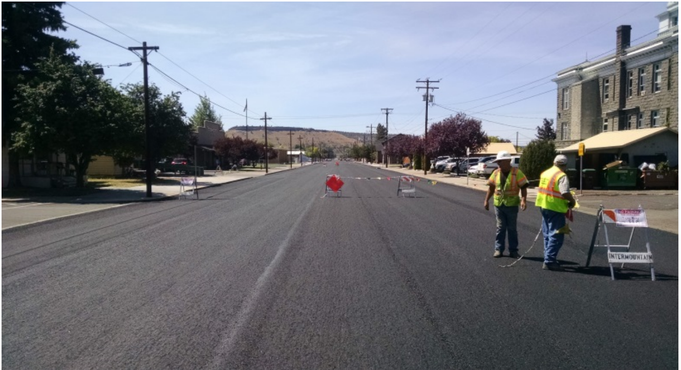
Seal coat in progress on NE 2 nd Street.
