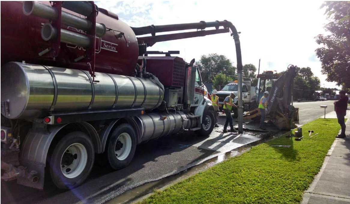
Public works staff installs a new water service.
