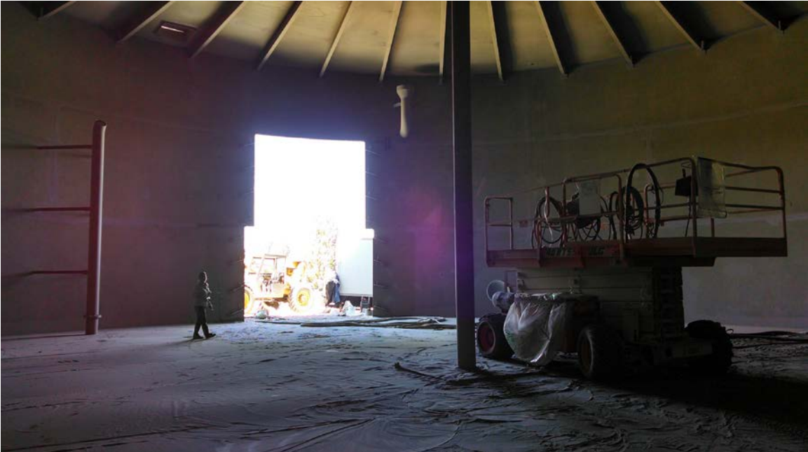
Construction progress of the Airport Water Tank #2.
