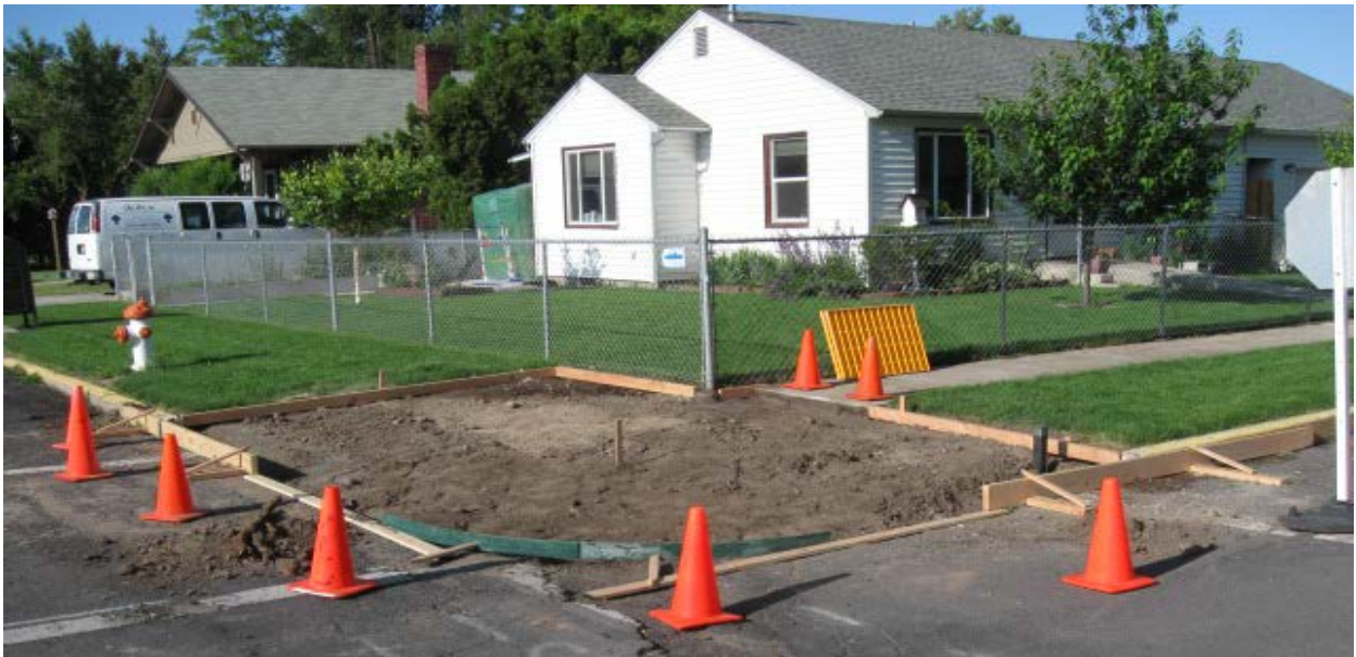
A street corner after the Transportation Department removed an old ADA ramp near a local school.
