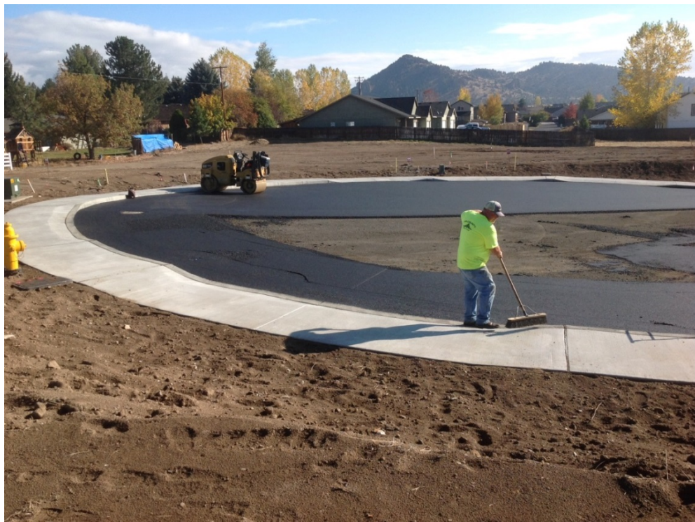
Contractors paving a cul-de-sac for a new development
