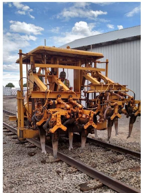
*Tamping and leveling a newly constructed yard spur at the Prineville Freight Depot.*
