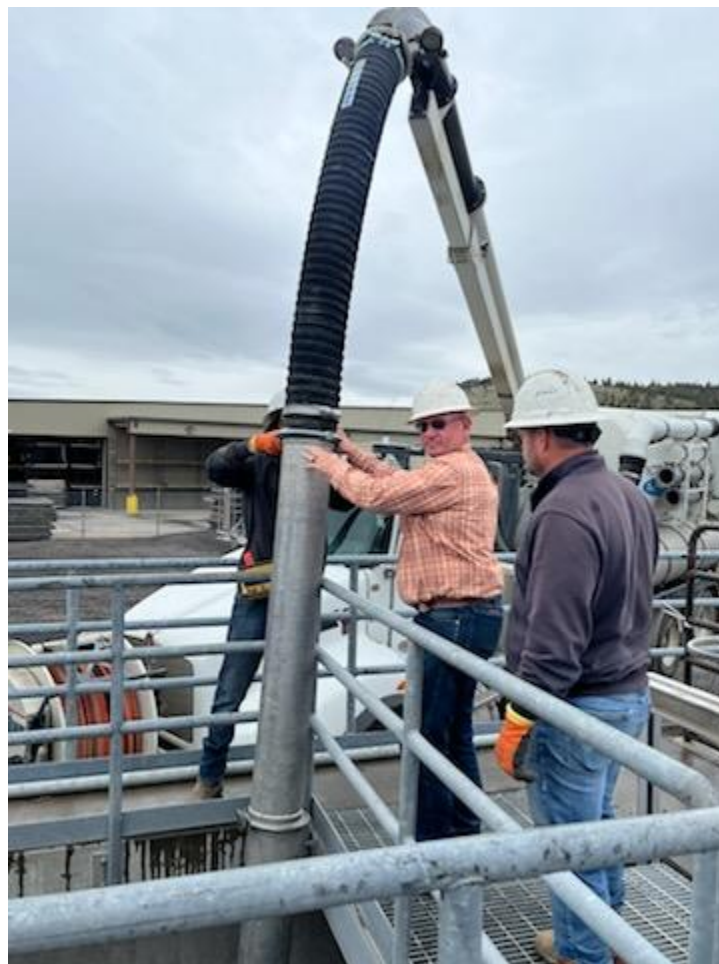
Wastewater work being done in April 2025
